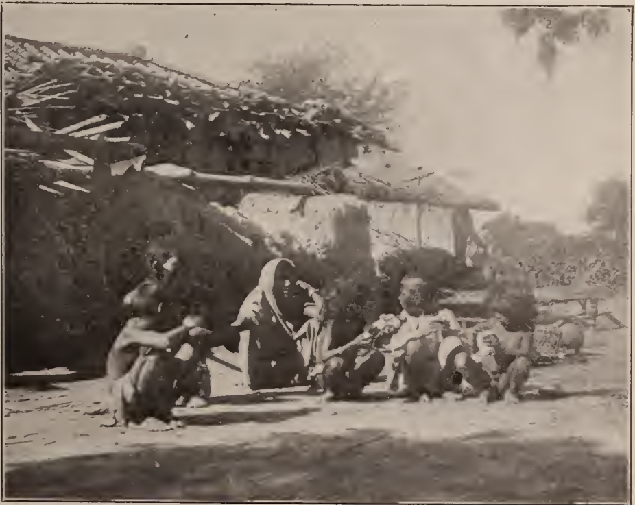
THE VILLAGE DOMS COMPLAIN THAT THEIR ROOF LEAKS
